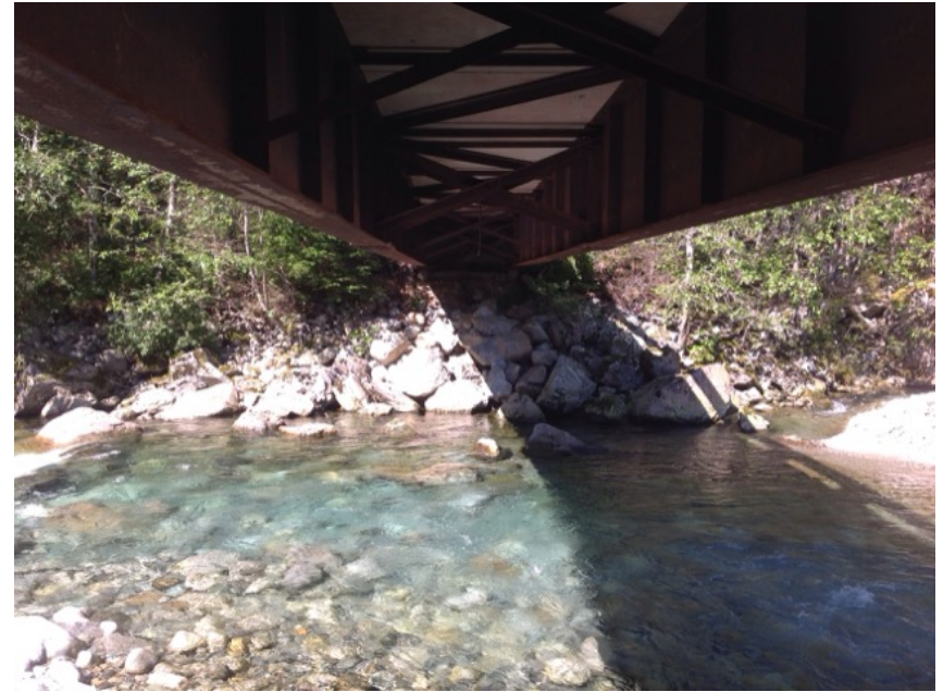
Right Bank Abutment when facing downstream
