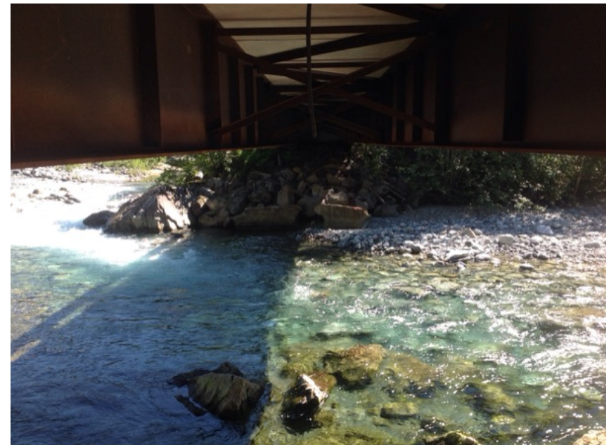
Left Bank Abutment when facing downstream
